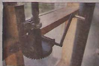
For less reliance on air conditioning, Calvino's design uses large screens that allow air to flow freely throughout the entire house. Above is a crank he designed and built to open and close the higher windows in the dining room, left. The crank is located against the wall of windows, behind the table.
