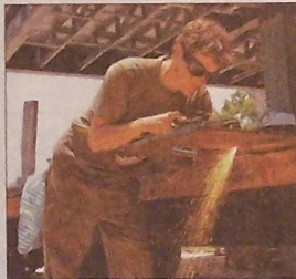
University of Florida student Brad Cooke, 19, cuts a piece of steel at the job site.
