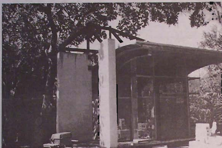
The roof and walls of the completed Ruskin guesthouse hang from 2 massive piers, much like a boat on a davit.
